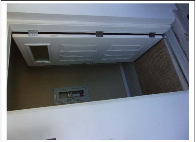
OPENING PROTECTION – The glazed front entry door is large missile rated. HarborSide Terrace Condominium Association FBC# FL17184.21 4280 Belair Lane, Unit C & D, Naples, FL 34103 03-22-2023
