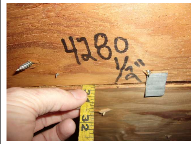
ROOF DECK THICKNESS – ½ inch plywood
