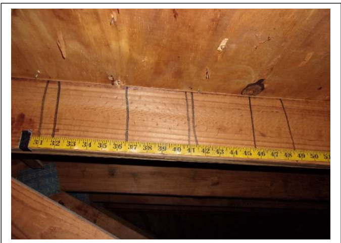
ROOF DECK ATTACHMENT – 8d nails within 6 inches in the field
