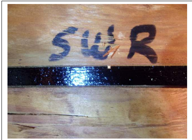
SECONDARY WATER RESISTANCE – A polymer adhesive (peel & stick) SWR Barrier was installed in 2021
