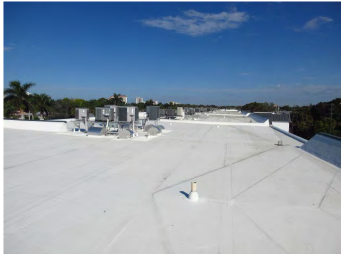
GENERAL VIEW OF ROOF COVERING
