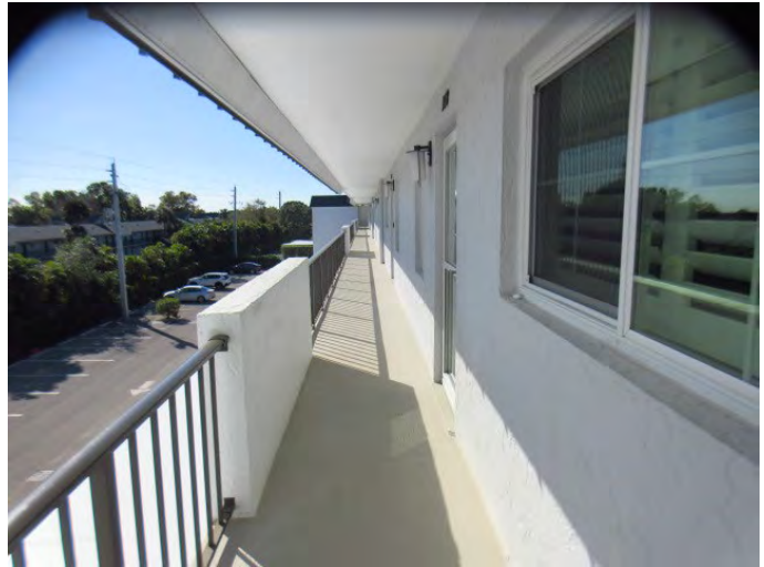
VIEW OF ELEVATED WALKWAY
