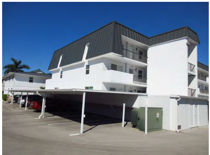
VIEW OF MANSARD ROOF
