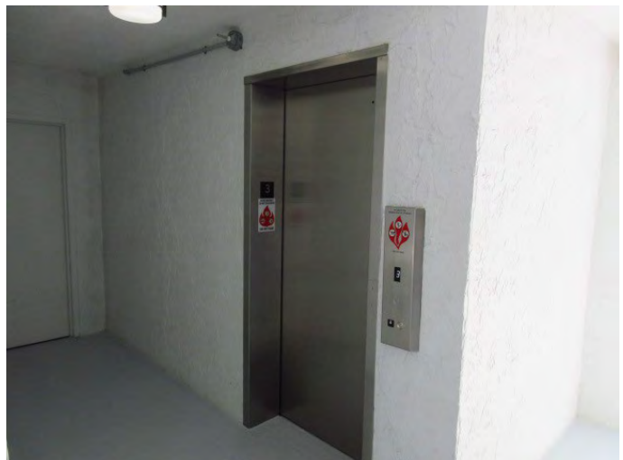
VIEW OF ELEVATOR LOBBY
