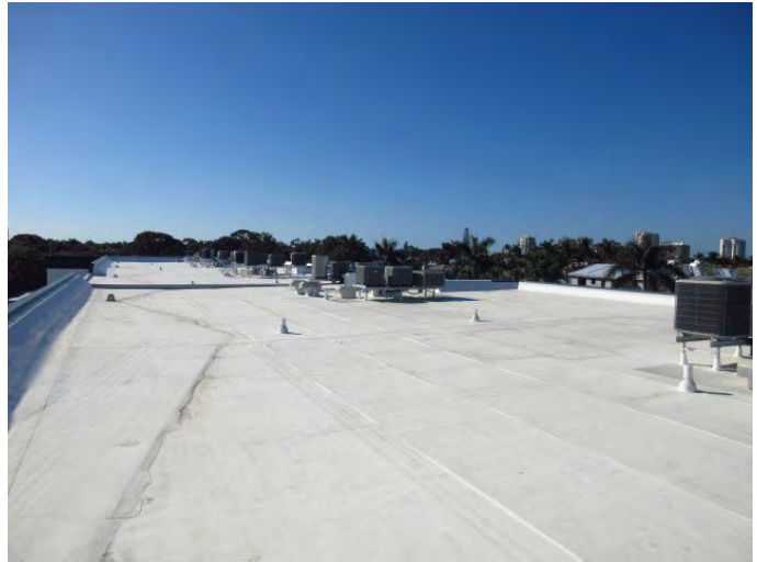
GENERAL VIEW OF ROOF COVERING
