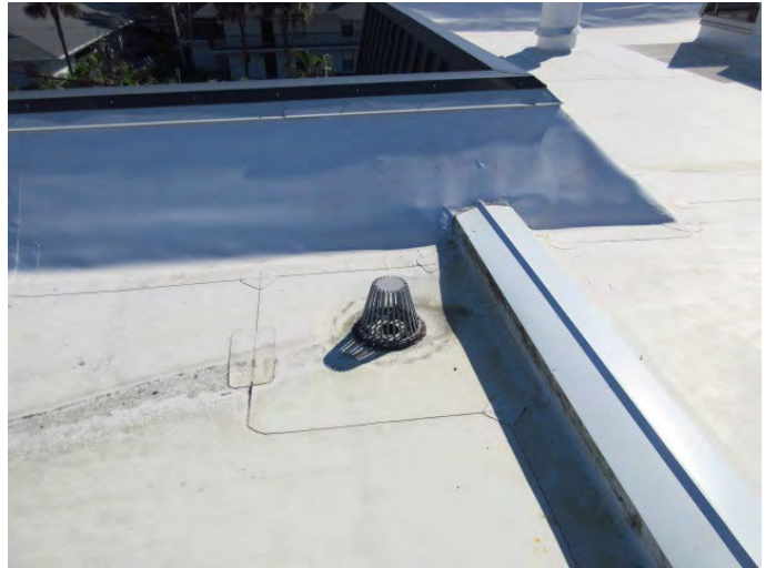
GENERAL VIEW OF ROOF DRAIN
