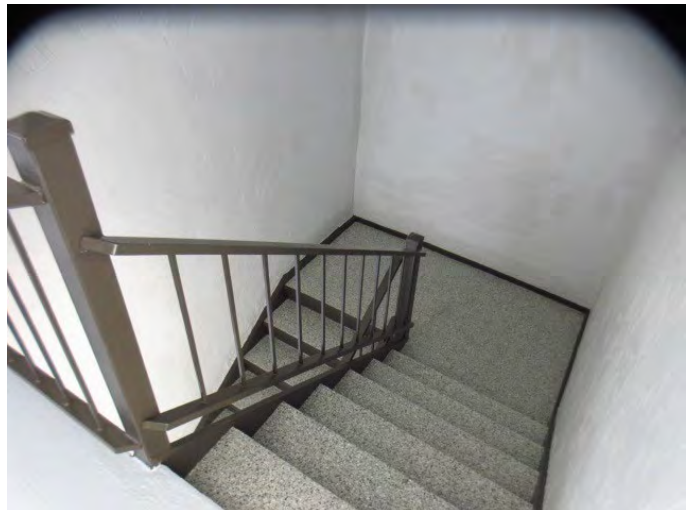
VIEW OF STAIRS
